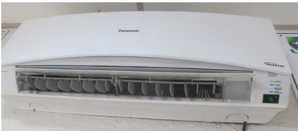
All window ACs are replaced with Inverter AC
